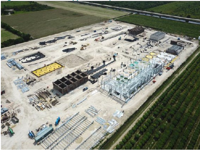
Figure 15: Atlantic Sapphire US 'pre walls and roof'
