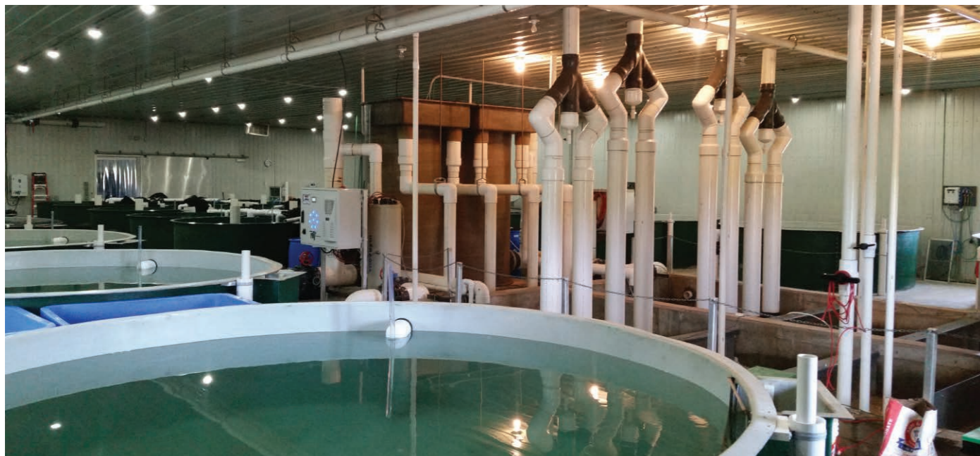
Interior of R&D Hatchery, Rollo Bay, PEI
