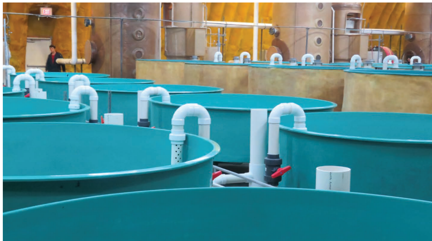
Early Rearing Tanks, Albany, Indiana.
